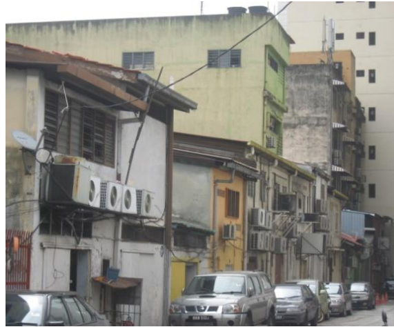
Figure 14: The lack of appropriate ventilation systems in shophouses
