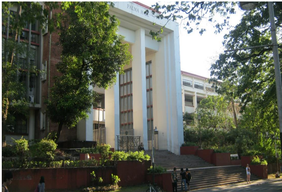
Figure 2 - The Arts and Sciences (AS) Building Steps serves as the main entrance of Palma Hall.
