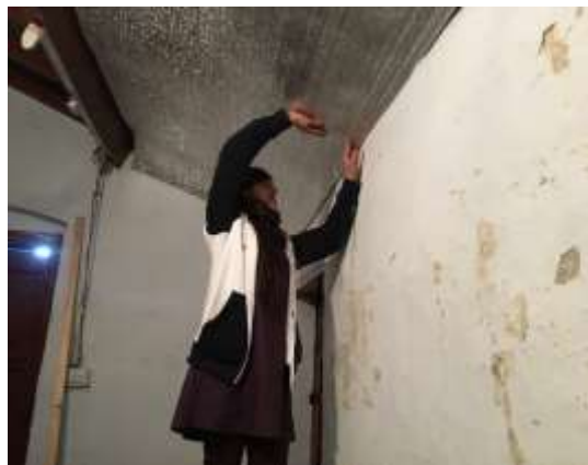
Figure 6. Application of PE Roll in T.R 2
