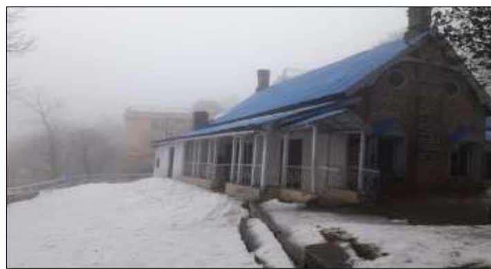
Figure 1. Exterior View of Test Building
