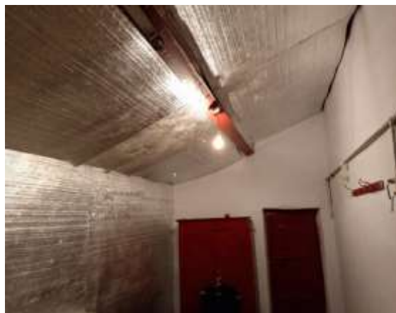
Figure 7. Application of PE Roll in T.R 2
