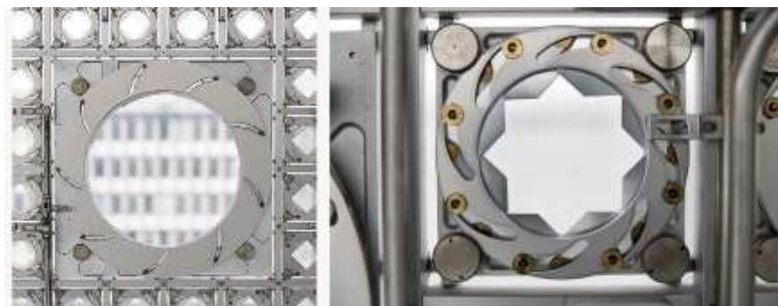
Figure 7. Images showing the details within the façade and its performance mechanisms at the Institut du Monde Arabe. Source: IMA., Cateloy, F. (n.d.).
